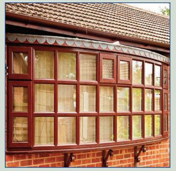
Bow windows are made of three to six windows that are all the same size. This gives the design of the space the ability to have a more gradually curved look and feel than the bay design, which has a sharper angle.
